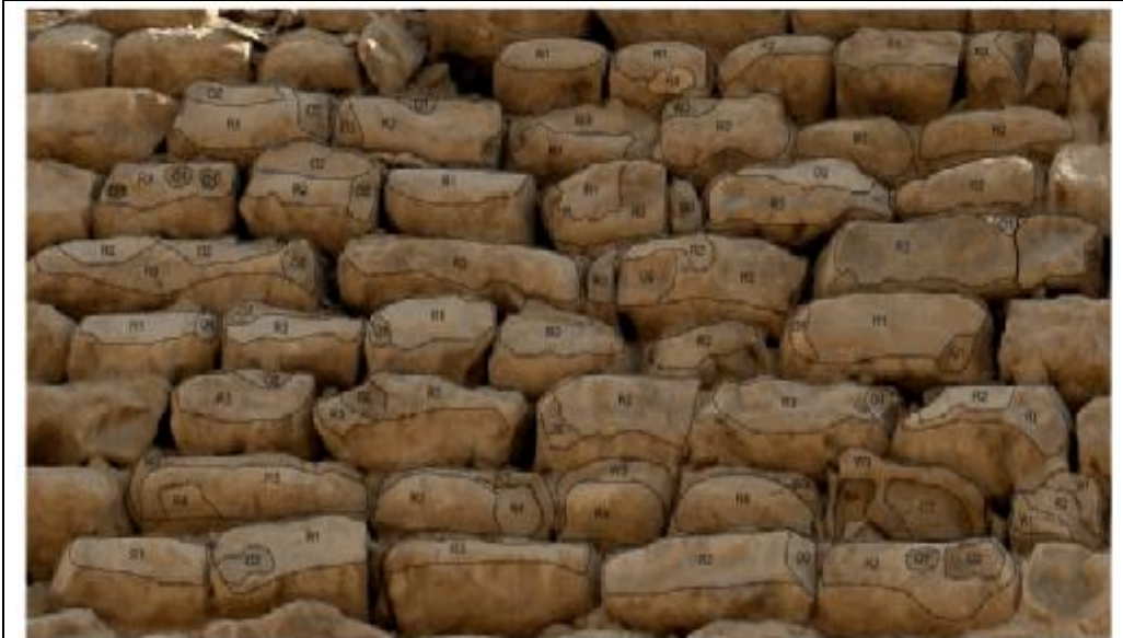
Rietumu fasādes parauglaukums. Sample area of the western facade.
