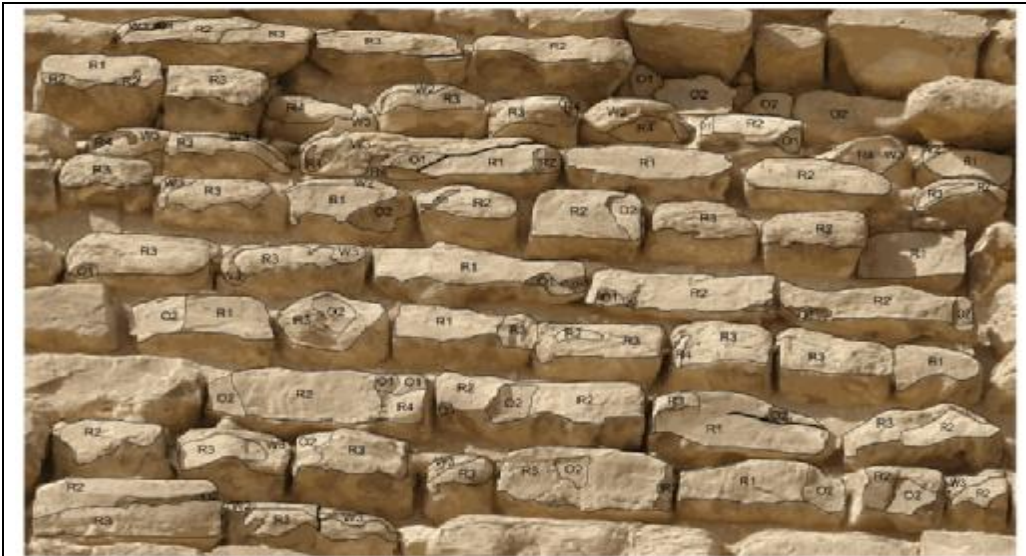
Austrumu fasādes parauglaukums. Sample area of the eastern facade.
