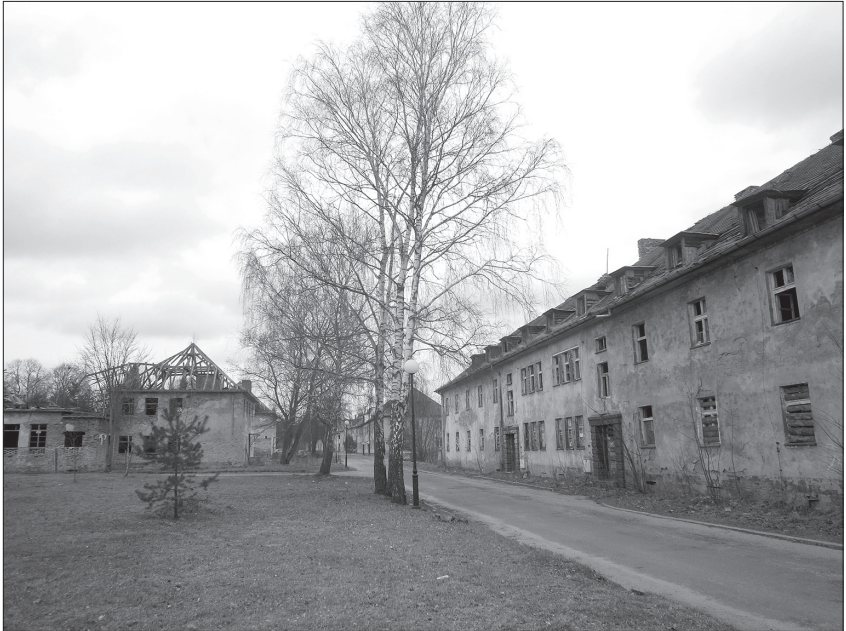
Fig. 1. Unrestored buildings. 2015. Photo by Dominika Czarnecka
