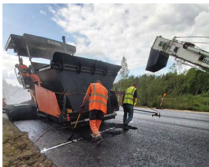
Fig. 1. FBG strain and temperature sensor integration into road pavement
